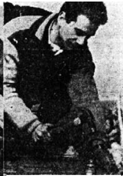
— Underfloor heating cables, similar to the ones used in the Mound "blanket," are fitted before the concrete floor is laid on top. There are no open fires in the building, and power plugs are fitted in each room. Two refuse chutes run from the top of the building for rubbish disposal.
