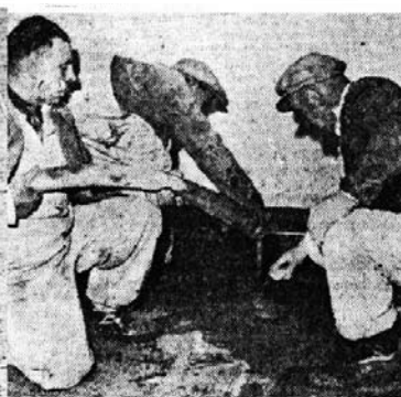
— Concrete floors being piped in from ground level—one of the ways in which machinery is speeding up the building work.
