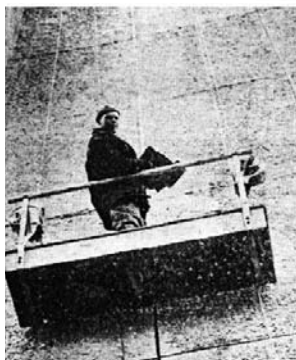
— Pointing the spaces between the pre-cast slabs is a lonely job for Otto Netz.
